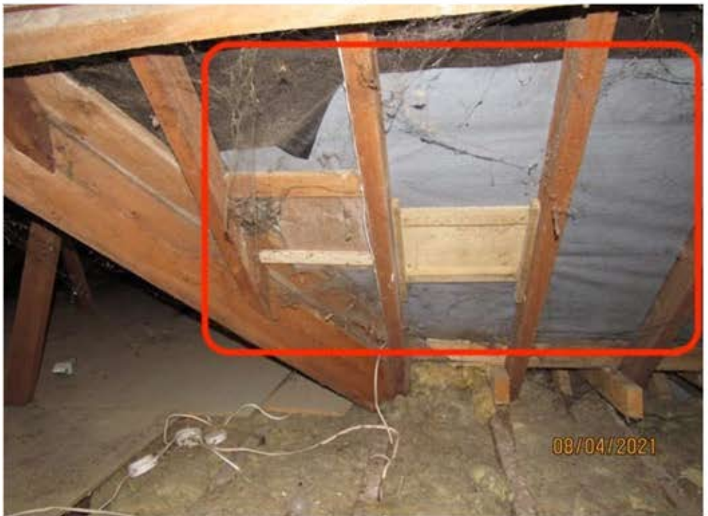
Patch repairs to east central slope
