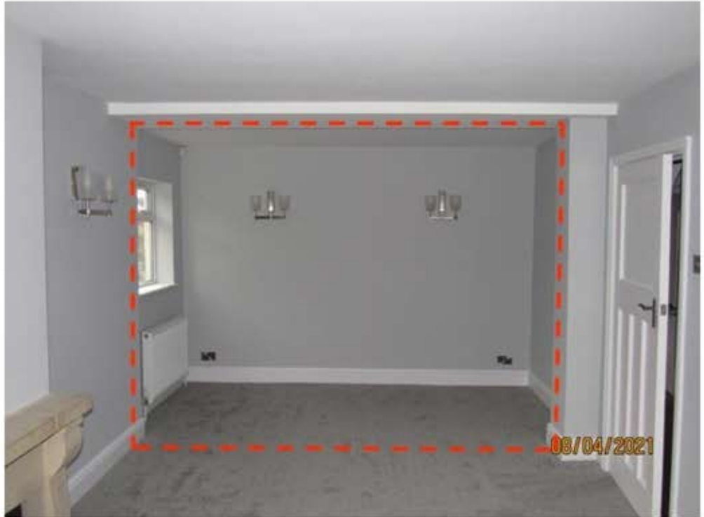
Position of wall removal in sitting room
