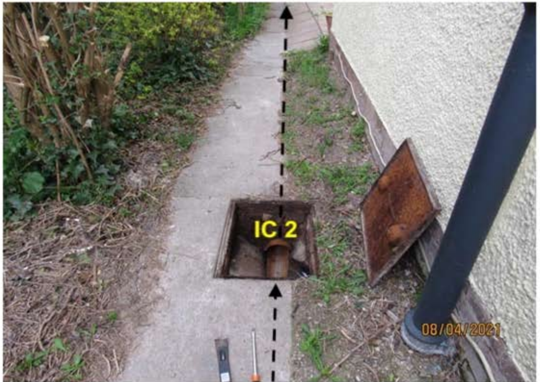
Drainage inspection chamber near east wall (IC 2)
