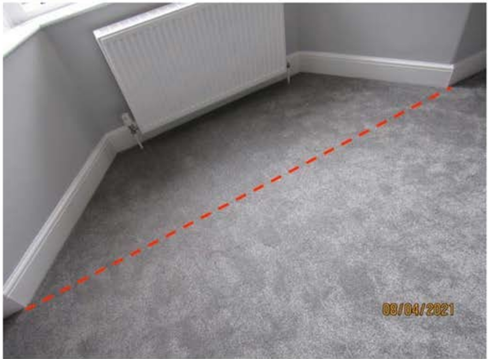
Floors of bay windows are timber
