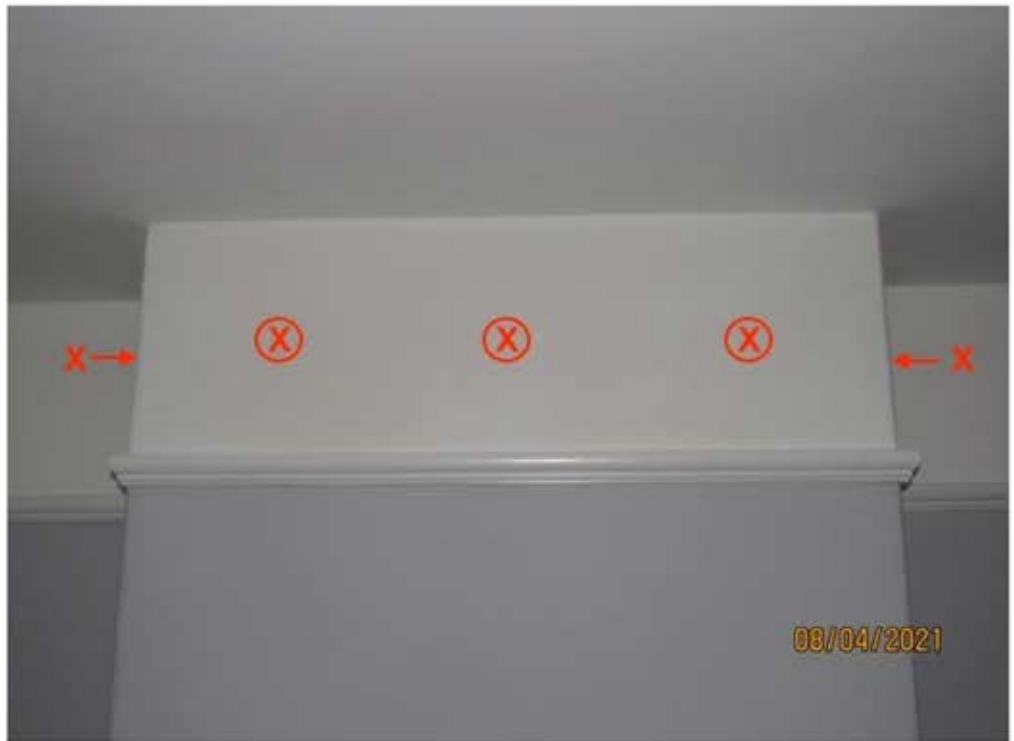
Moisture meter readings in bedroom 2 (High = red X within red circle. Above average = red X)
