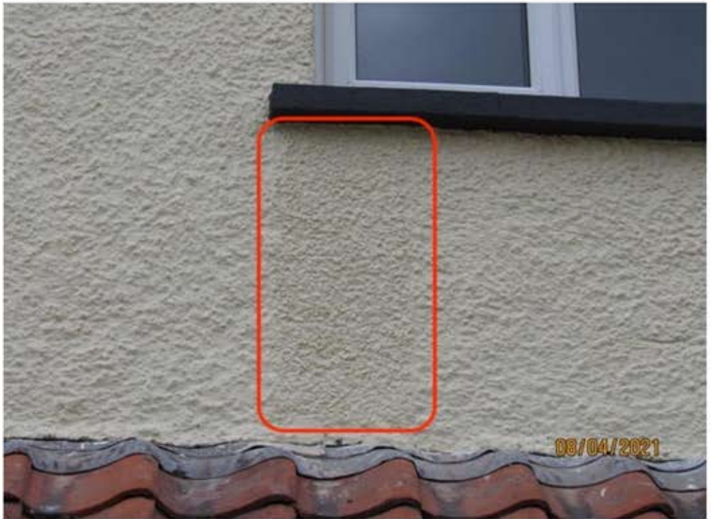
Example of different render used for repair work
