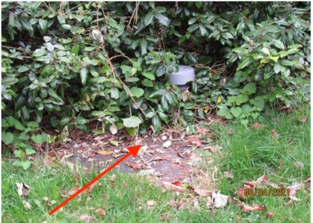
Estimated position of septic tank in garden
