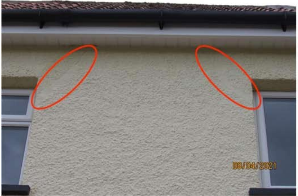
Areas of repair above windows on south wall
