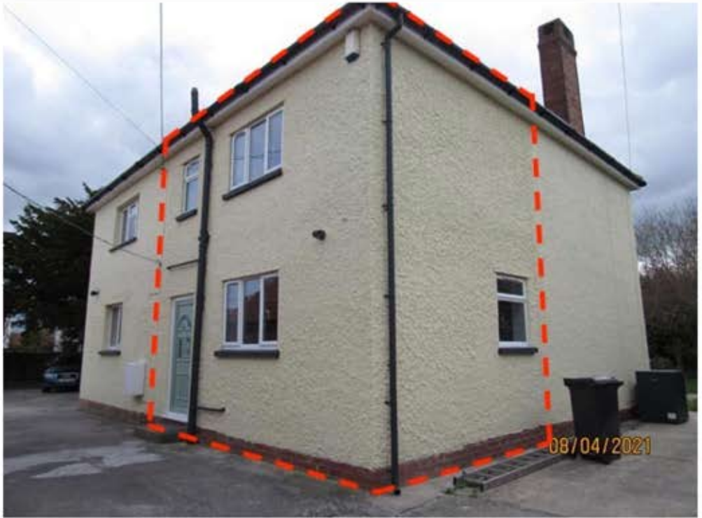
North and west elevations showing corner extension
