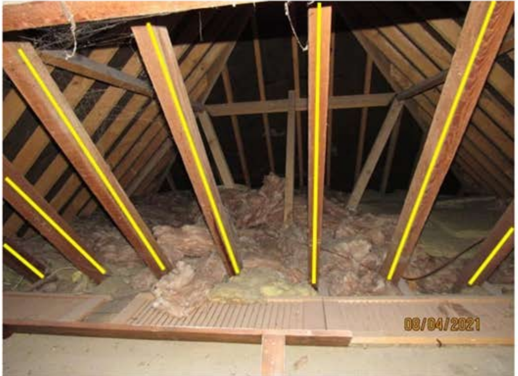
View of north-west extension with yellow lines indicating original roof rafters
