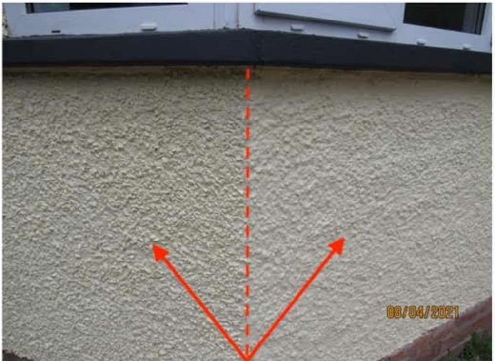
Different renders applied to walls below west bay window
