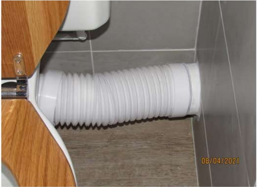
Flexible pan connector in ensuite
